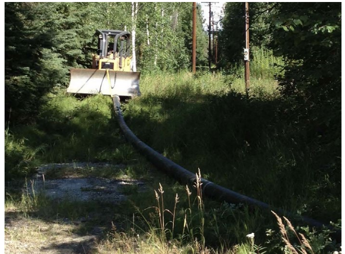
Pipe being pulled through narrow easement
