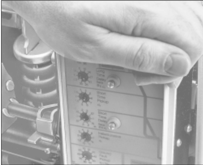
7. Lower trip unit onto support plate.
