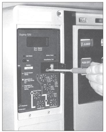
Figure 3. Installation of the Rating Plug and Mounting Screw
