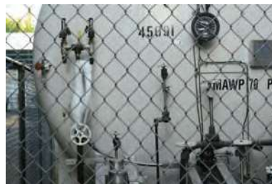
Difficult inspection sites
