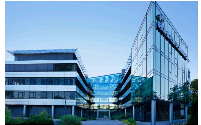
Rohde & Schwarz headquarters in Munich, Germany.
