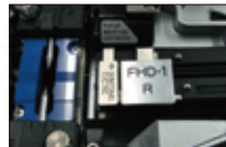
Drop cable splicing with fiber holder system
