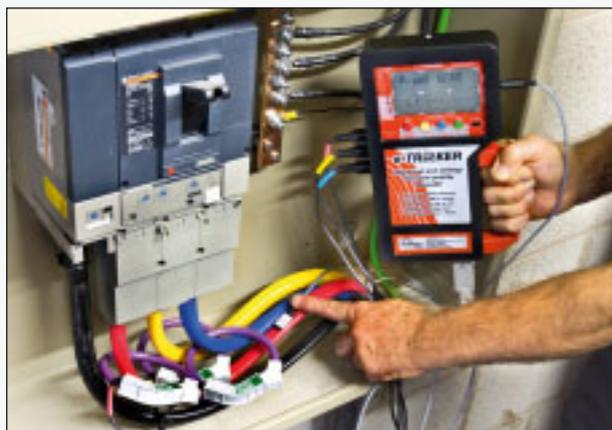
**Pulse interface** (option) The battery operated isolated interface unit enables Tracker to record volt free pulse outputs from water, gas, electricity or optical meter readers, (Magpeye).
