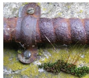
Figure 23. Cleaning up sources of PIM can cure interference problems
