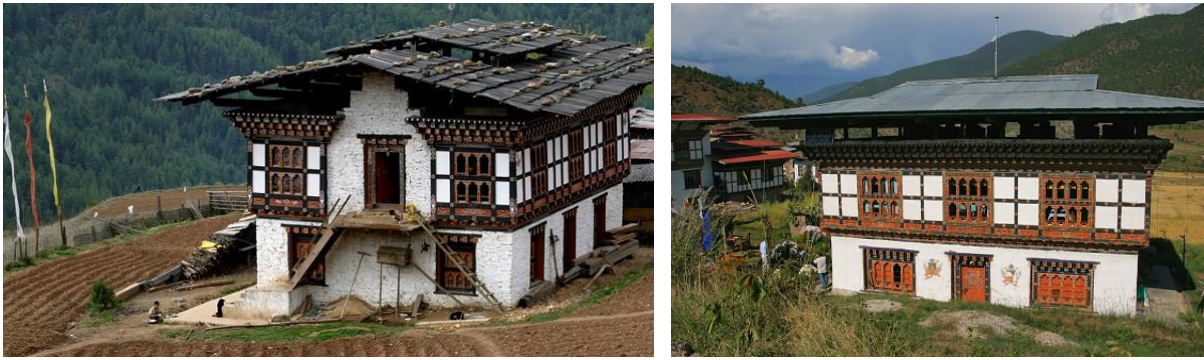
Fig. 1) Modern influences on Bhutanese society can also be found in its architecture. For example typical wood shingle roofs weighed down with rocks (left) are replaced with low maintenance corrugated sheet roofs (right). Image credit: Bhutan Nuns Foundation; Living Travel.
