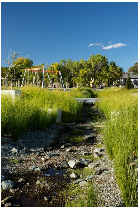
Figure 12: Green multi-use detention area (Landzine, n.d.)
