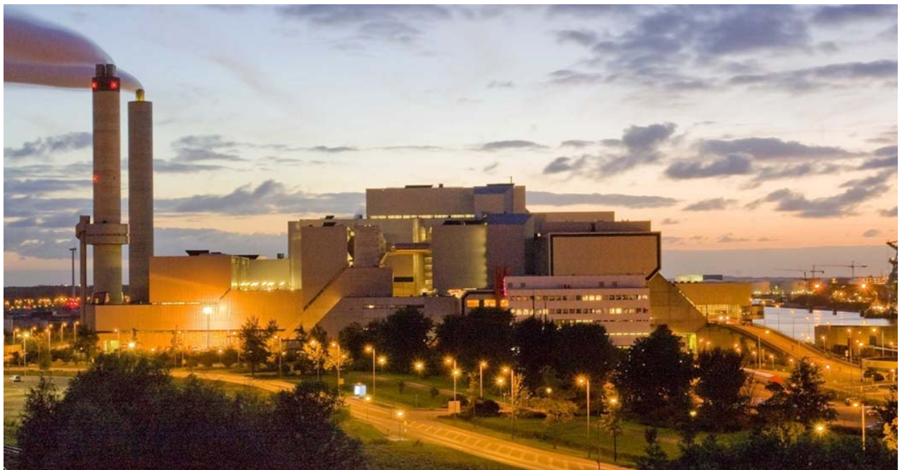
Figure 1: The waste to energy plant in Amsterdam
