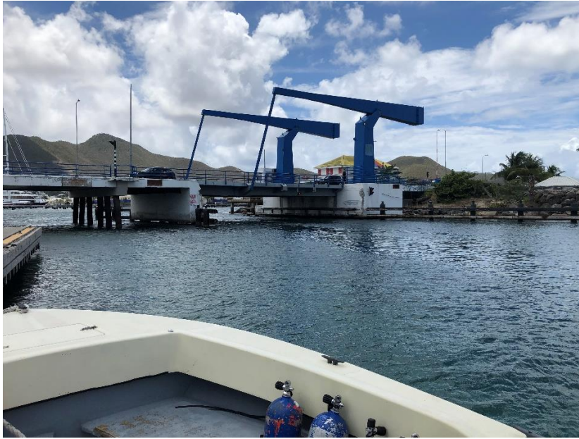
Figure 54. Bridge Channel water testing site.
