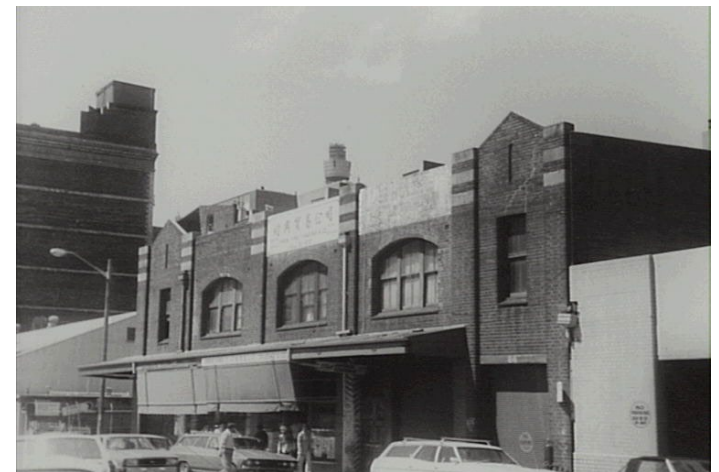
The family general store on Harbour Street
