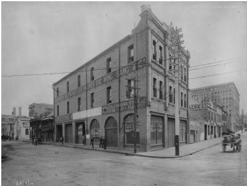
The warehouse building of Wing Sang & Co in Haymarket, Sydney (c1910)
