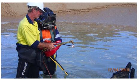
*Figure 9. Lighting the thermal lance in preparation for cutting, facing S.* (Cosmos Archaeology. 17<sup>th</sup> April, 2015).
