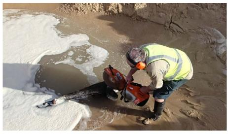
*Figure 21. Cutting of the bow section with hand held circular saw, facing S.* (Cosmos Archaeology, 17<sup>th</sup> April, 2015).
