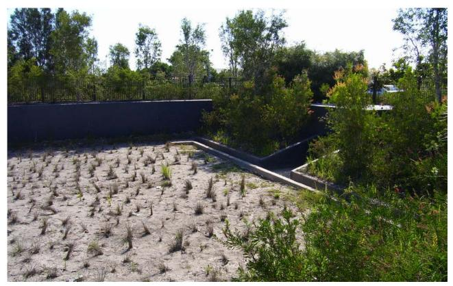
Figure 2 Poorly integrated bioretention basin (source: Switchback 48 Consulting)
