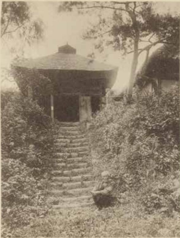
Fig. 42. The Kannon Temple at Kamahara, built before the Tenmei period. The front stone stair, which consisted originally of 120 steps, had the lower 105 buried by the Volcanic Avalanche of 1783, there remaining since then only 15 steps.
