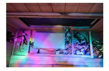
Once exposed, remove the Phillips screws anchoring the power box to the ground - two on the long front edge and one on the right edge close to the back wall (as you are facing the back wall).
