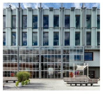
PPG supplied PPG *Duranar* SUNSTORM® coatings for 500 interior metal panels that are visible through a series of stacked 20-foot-tall light boxes that comprise much of the building's façade.
