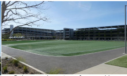
Solar panels on top of our parking structures surrounding our central park
