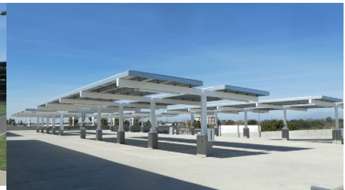
Solar panels in our newest parking structure
