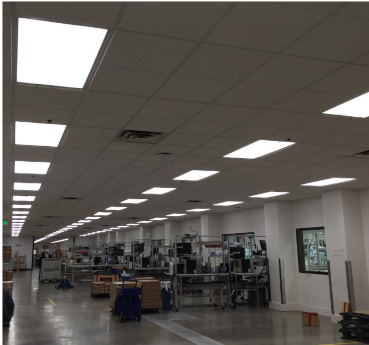
LED Lighting Upgrade Project
