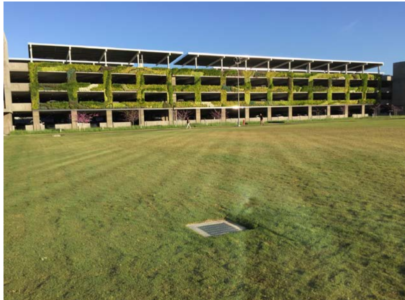
Two 30,000 gallon underground storm water harvesting tanks in Irvine’s Central Park
