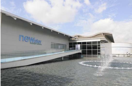
NEWater Visitor Center, Singapore
