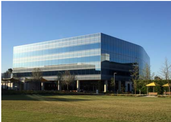
LEED Gold Certified Edwards Headquarters Building, Irvine, CA
