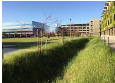
Natural Bioswales for Storm Water Filtration
