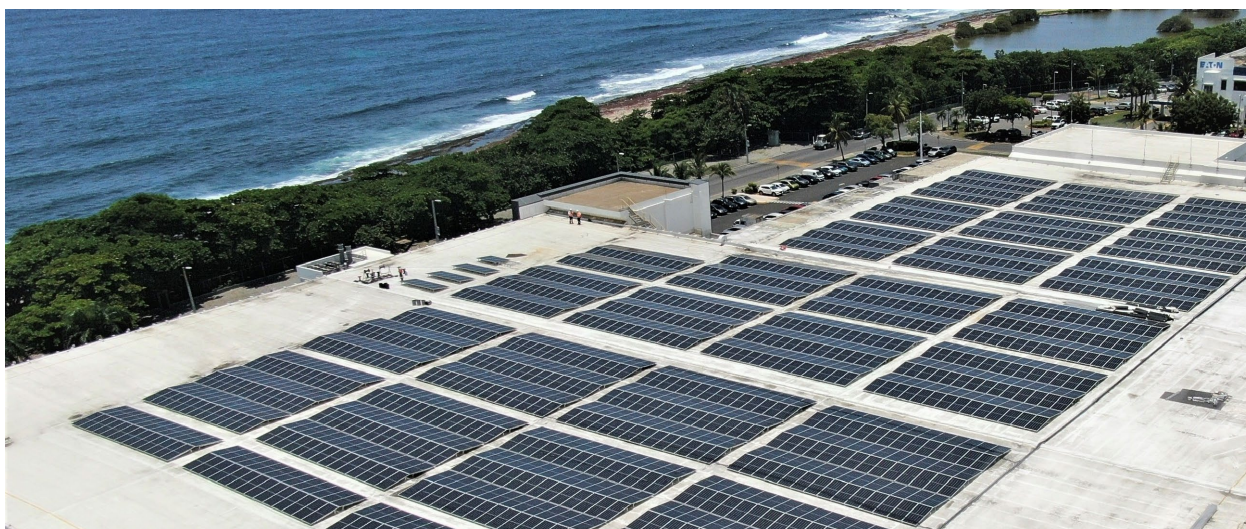
A 1 MW solar panel project is currently underway at the Dominican Republic manufacturing plant, which will provide renewable energy and reduce the plant's overall GHG emissions by 15%.
