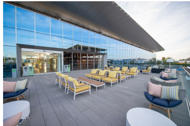
Rooftop view from our new LEED-certified Café & Conference Center in Irvine, California.
