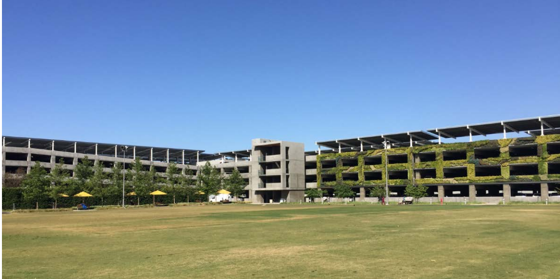
Solar Photovoltaic Panel Electricity System, Top of Parking Structures, Irvine, CA
