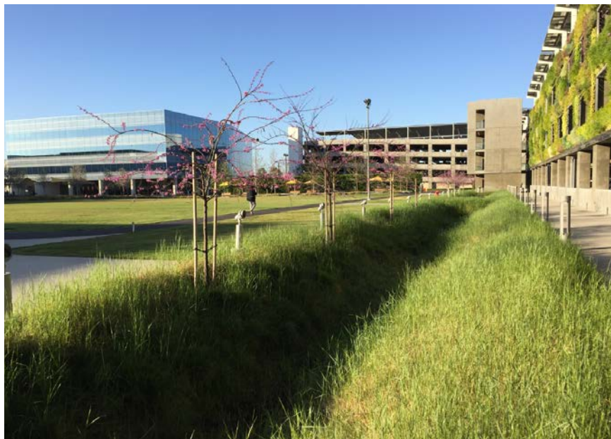
Natural Bioswales for Storm Water Filtration
