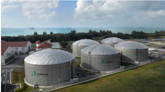
Singapore’s sembcorp NEWater treatment and storage facility
