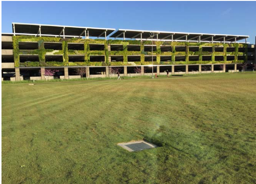
Two 30,000 gallon underground storm water harvesting tanks in Irvine's Central Park
