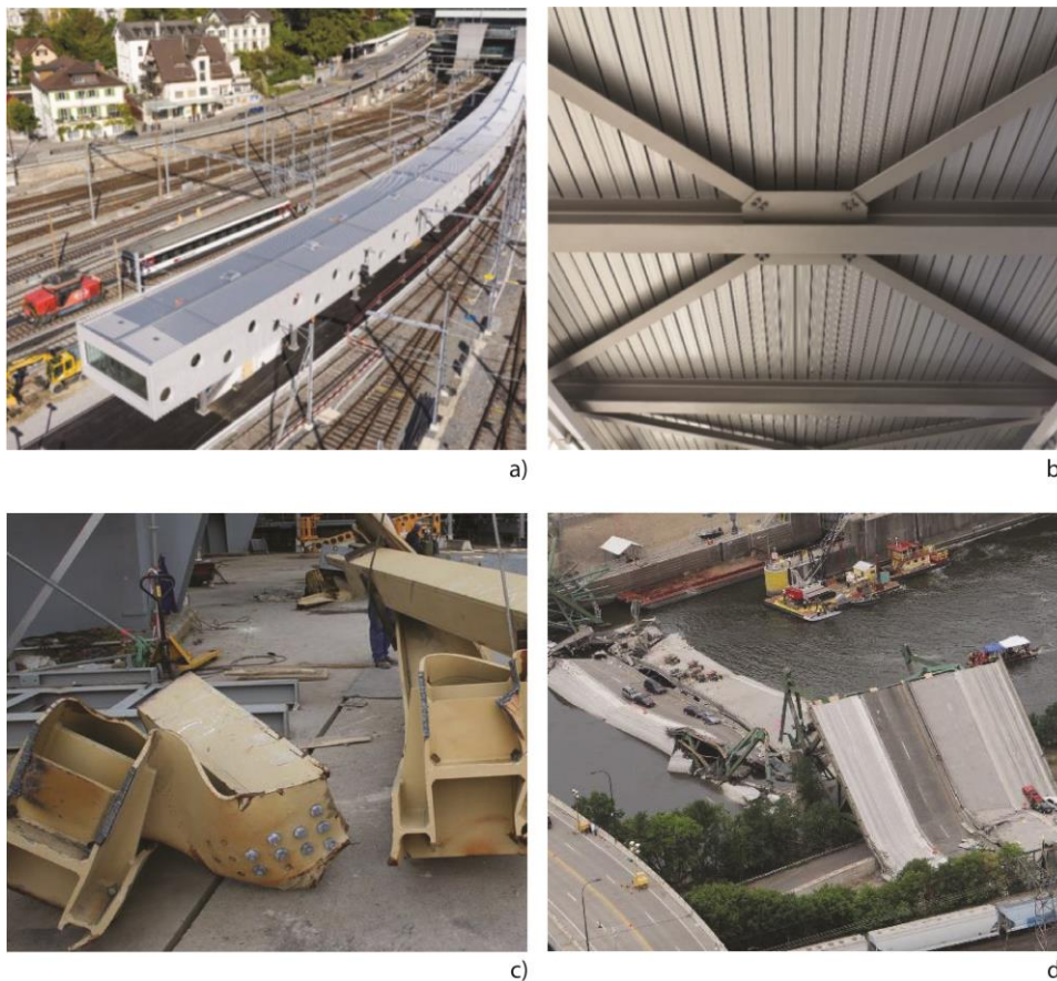
Figure 1: a) Gateway at Bern railway station; b) typical gusset plate connection [1]; c) Collapsed scaffolding from Neurath Power Station [2]; d) Collapse of the I-35W Mississippi River bridge [3]
