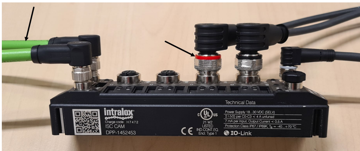
Figure 7: Cable connections and color coding
