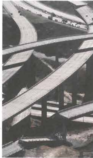
Above: A freeway interchange shatters from the impact of the Northridge, California earthquake, 1994.
