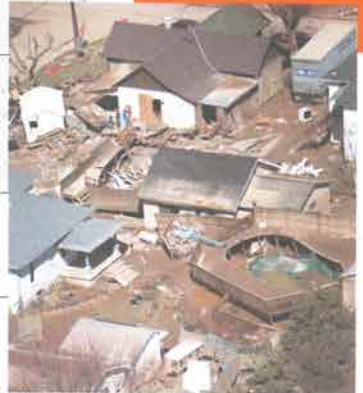
Floodwaters damage houses, swimming pools and storage sheds in Falmouth, Kentucky, 1997.
