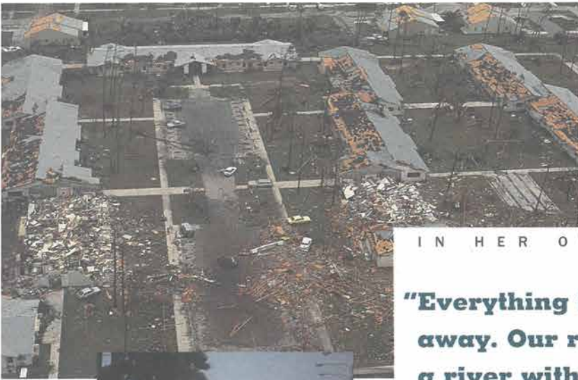
Left and bottom: Damage caused by Hurricane Andrew, Florida, 1992.
