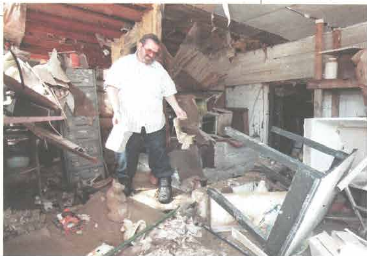
A homeowner sorts through the waterlogged remains of his basement hobby room, which was completely underwater in Silver Grove, Kentucky, 1997.
