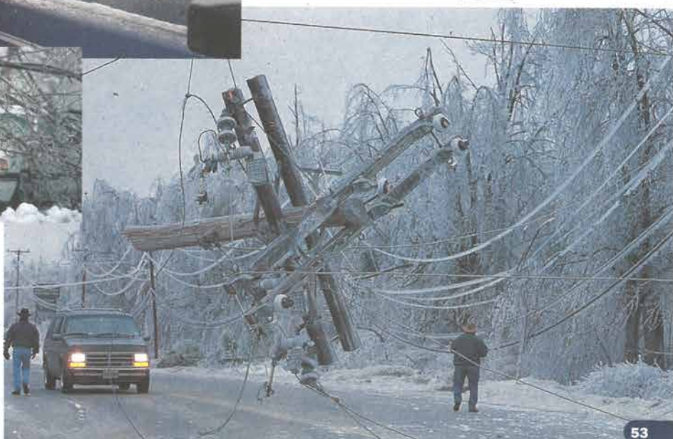
Below: Ice-covered power lines snap a utility pole in half and shut down traffic on this road in Maine during the 1998 ice storm that hit New England and Canada.
