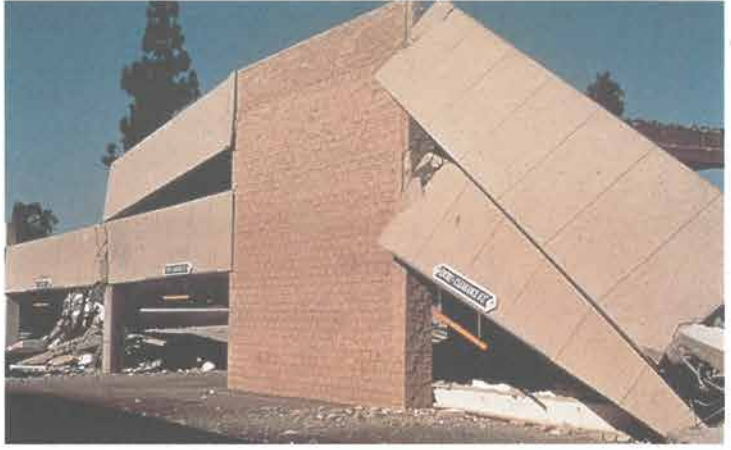
The 1994 Northridge, California earthquake causes six precast concrete parking garages to partially collapse.
