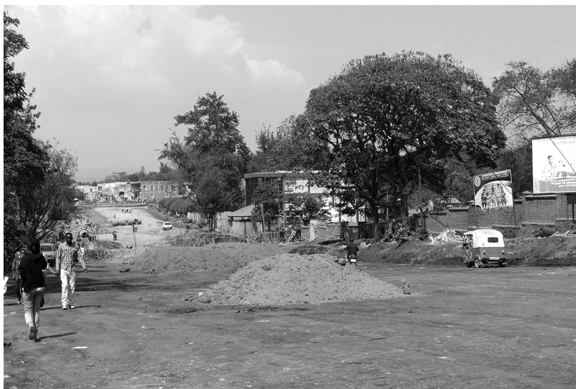
FIGURE 1.2. Road construction in Jimma. Photo by Alise Osis.
