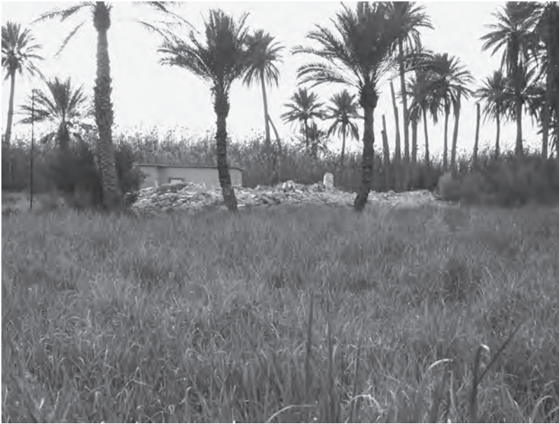
1.2. Hameed's rebuilt house behind its bombed form. His newer date palms foreground the decapitated trunks of dead ones. Photo by Kali Rubaii, 2023.
