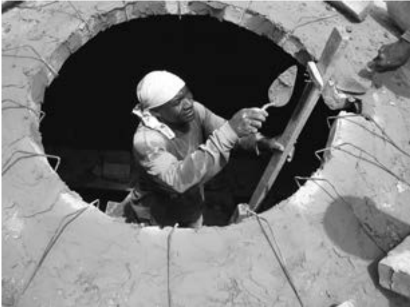
Figure 1.8. Large-scale biodigester under construction, 2011 (Photo by Brenda Chalfin)
