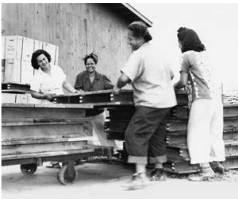
FIGURE 1.2 · From back of print: “Isabel Nascimento ( back left ), Catherine Ohumukini ( right ), Harriet Garcia ( front left ), and Sally Young working on pallets. (Scene at store-house).” United States Navy ?, undated. Hawaii War Records Depository HWRD 2164, UHM Library Digital Image Collections.
