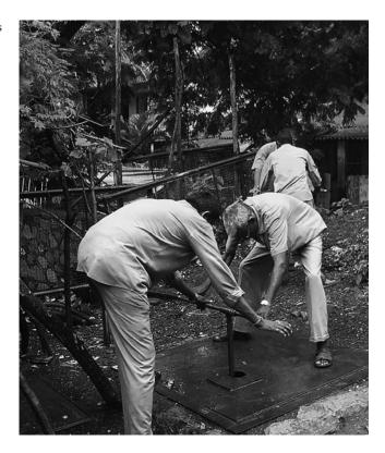
because the amount of water the city gets every day is finite and materialized by valve operations, to give one hydraulic zone more water is also to give another zone less.
