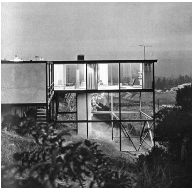
1.6 Smith House, Case Study House No. 16, Los Angeles, California, 1958. Craig Ellwood Associates, architects. Photograph by Marvin Rand. Marvin Rand Archive, College of Environmental Design, Cal Poly, Pomona.
