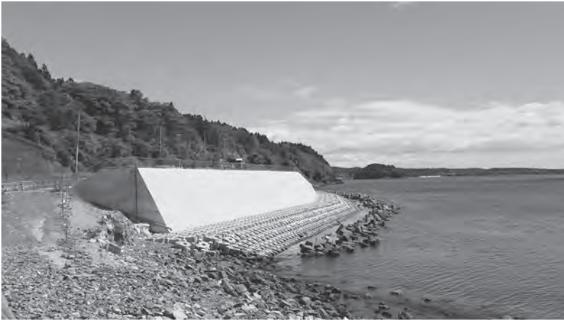
FIGURE 1.3 A seawall facing Shizugawa Bay.
