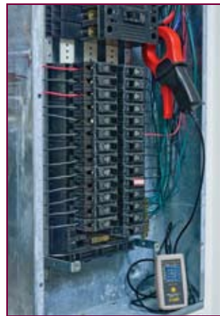
L101 recording branch circuit current.
