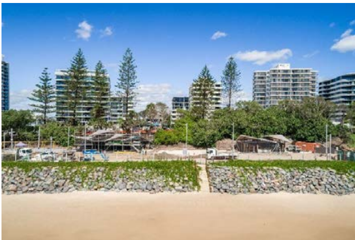
Figure 3 New beach stairs, BBQ Shelter and Public Amenities building under construction
