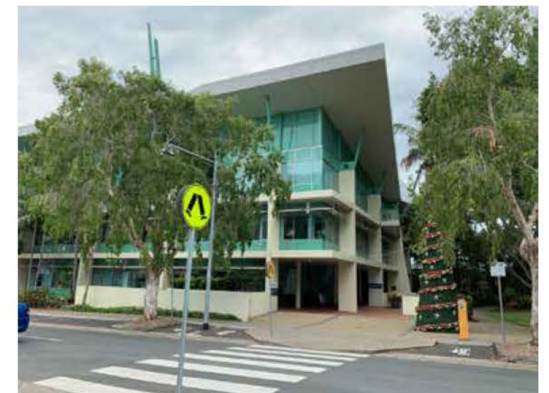
Caloundra Administration Building 2019
