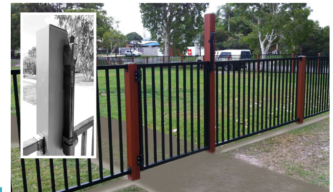
Figure 20: Typical playground / play space pedestrian gate (inset: magnalatch or equivalent) (for guidance only – site specific design required)
