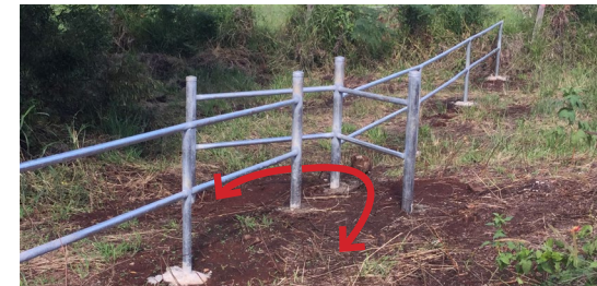
Galvanised post and rails in a 'u' shape
