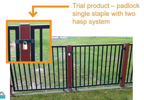
Figure 23: Typical vehicle gate (inset: two lock system) (for guidance only – site specific design required)
