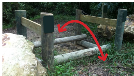
Timber post and step over
