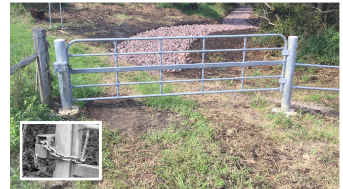
Figure 3: Vehicle access gate 'super heavy duty' (inset: lock system) (for guidance only – site specific design required)
