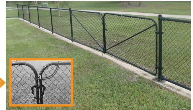
Figure 18: Typical vehicle access gate for DEA (inset: lock system) (for guidance only – site specific design required)
