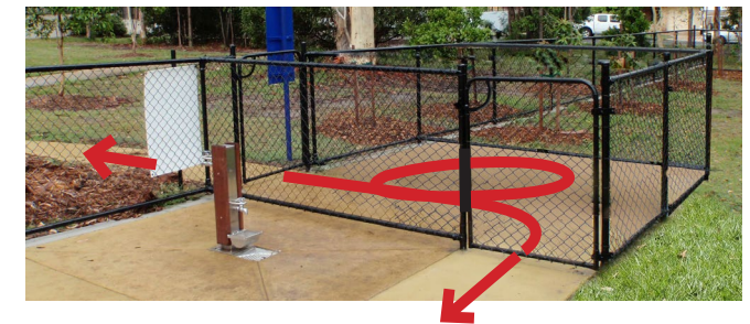
Figure 16: Typical standard pedestrian gate for a dog off leash dual gate entry (for guidance only – site specific design required)
