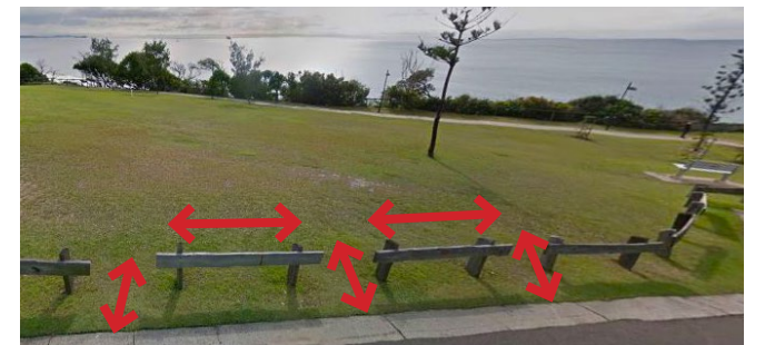
The gaps between barriers allow entry / exit and reduce pedestrian speed
