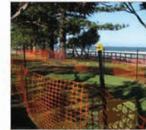
TREE PROTECTION FENCE - SAFETY BARRIER MESH
