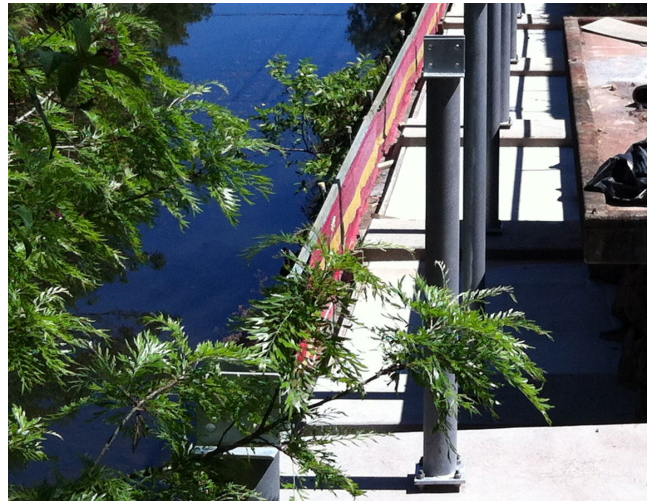
2: HDG steel posts bolted to footing
