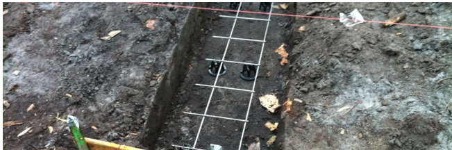
1: Boxing and reinforcing for poured in-situ concrete footings
