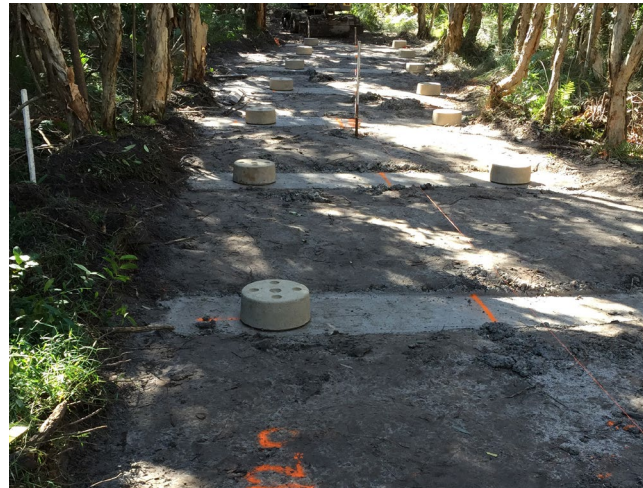
2: Precast concrete stump on poured in-situ footings to support bearers
