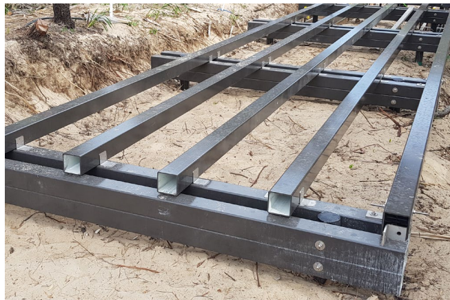
4: FRP joists stainless steel angle bracket fixed to FRP bearers
