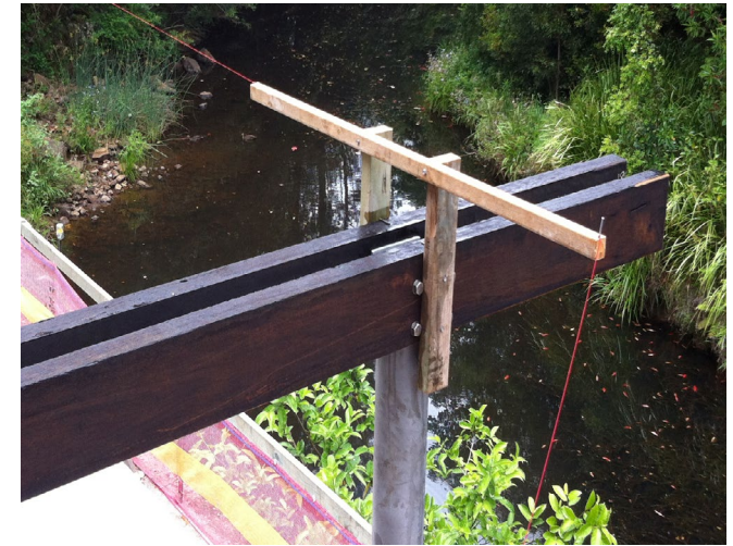
3: Double timber bearers (headstock) bolted to steel post
