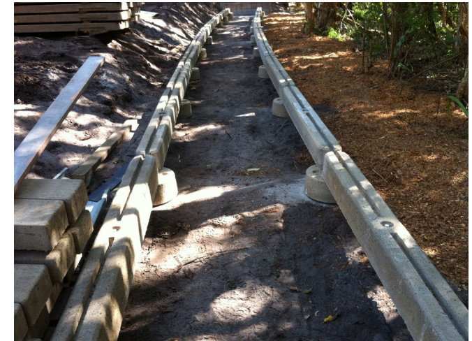
3: Precast concrete bearers mounted on stump units
