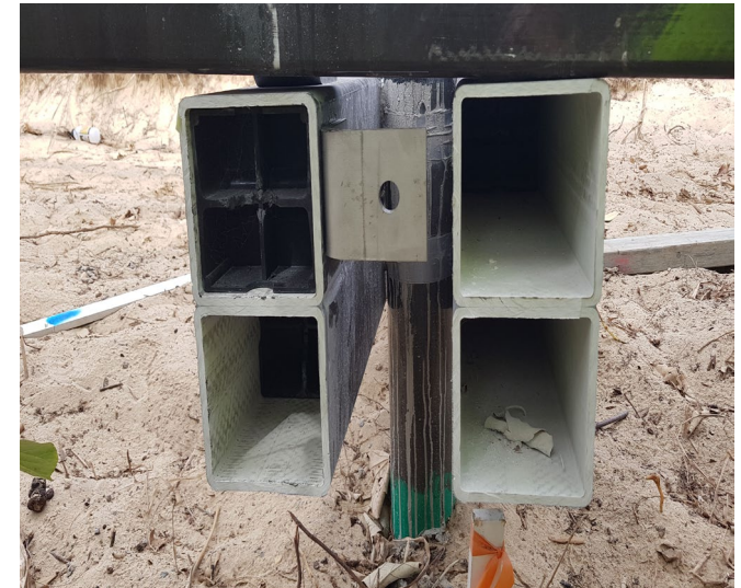
3: Double FRP headstock bolted onto HDG steel screw piles (concrete core filled)
