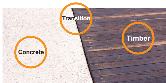
Figure 7: Typical timber to concrete pathway transition (for guidance only – site specific design required)
