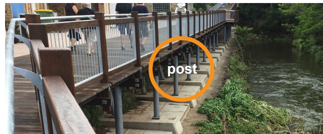
Figure 4: Example – posts of a boardwalk (for guidance only – site specific design required)
