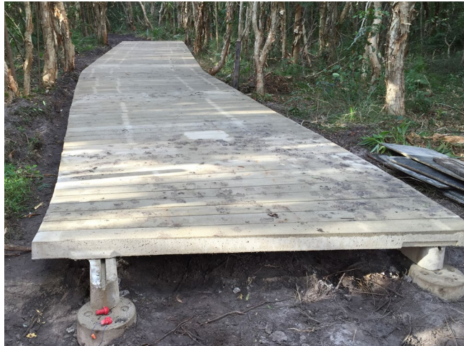
4: Precast interlocking concrete deck planks on bearers, secured into channel
