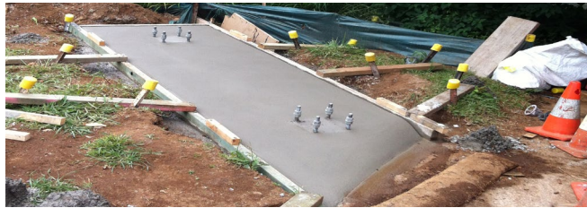
1: Boxing for concrete pad footing
