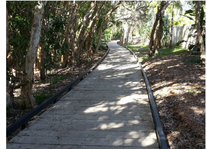
6: Recycled plastic kerbs (edge restraint) plus spacer blocks
