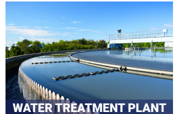
WATER TREATMENT PLANT
