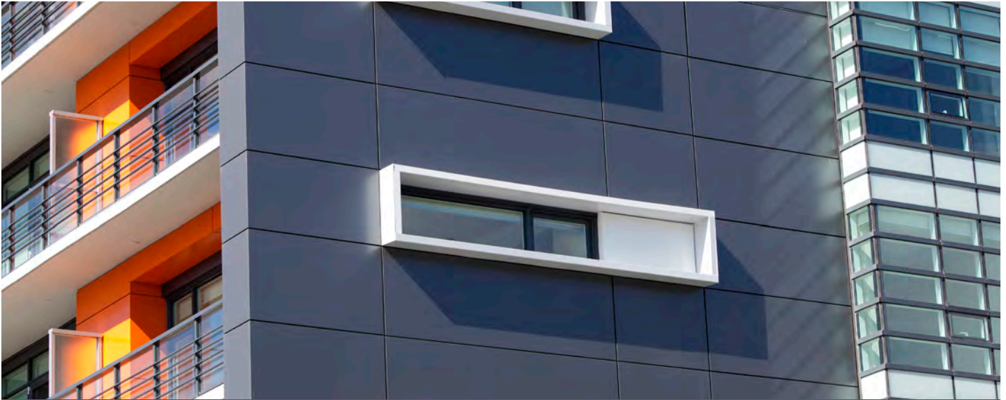
Cladding made from coiled aluminum is another emerging use for energy-curable coatings.
