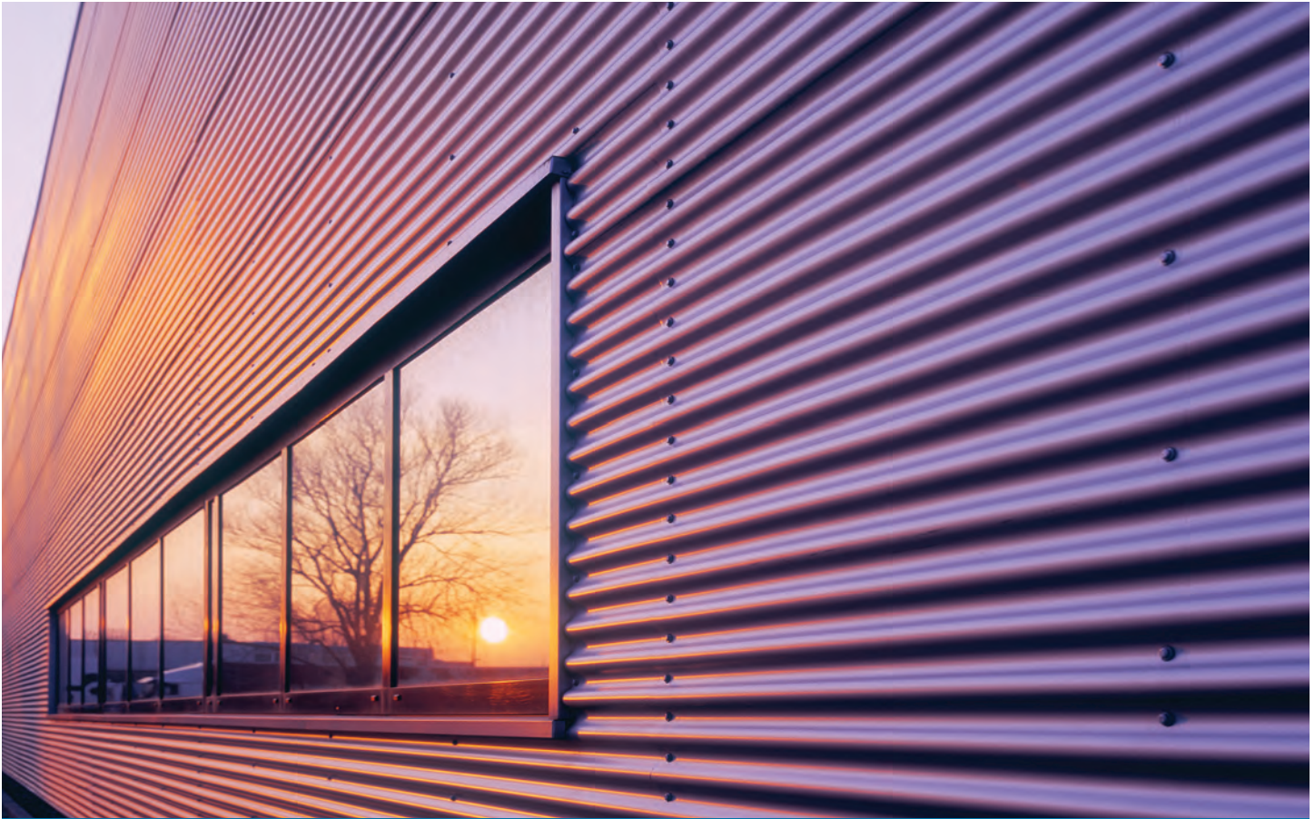
Architectural panels made from coiled aluminum is one of the many emerging uses for energy-cured coatings.
