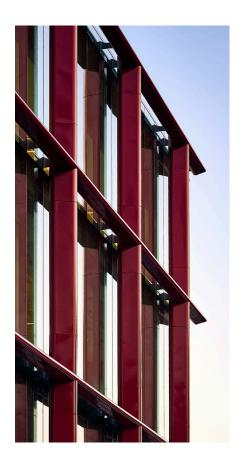
it was top-coated with the high-gloss powder. By inserting a bake interval between the application of the base coat and the topcoat, Spectrum's coating system prevented the glass flake in the topcoat from bleeding into the base coat, which further enhanced the finish's three-dimensional effect.
