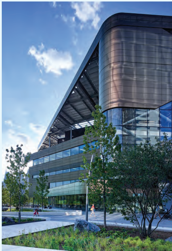
PVDF coatings used on a monumental building
