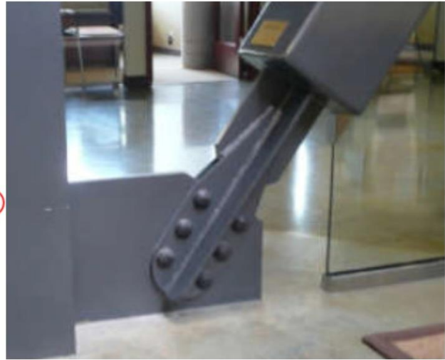
b) Image of Constructed Corner BRB Connection
