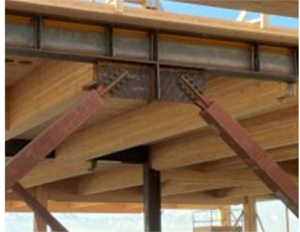
b) Image of Constructed Chevron BRB Connection
