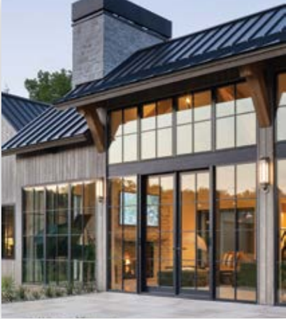
Photo © Architecture: Tommy Everson (Everson Architect) Builder: Gordon James Construction Photography: Jon Huelskamp | LandMark Photography
