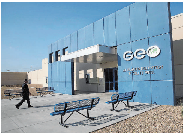
The Adelanto Detention Facility, shown in November 2013, houses an average of 1,100 immigrants in custody pending a decision in their cases or awaiting deportation.
